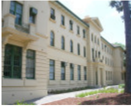
FORMER VICTORIA POLICE DEPOT SOHE 2008
