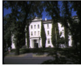
1 former Victorian police mounted branch depot St Kilda Road Southbank front entrance
