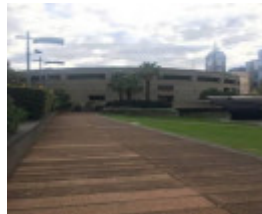
2019_Walkway rear of Forward Surge.jpg
