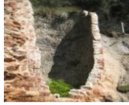
Bell Point Lime Kiln, September 2011
