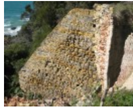
Bell Point Lime Kiln, September 2011
