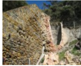
Bell Point Lime Kiln, September 2011
