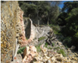
Bell Point Lime Kiln, September 2011
