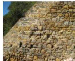
Bell Point Lime Kiln, September 2011
