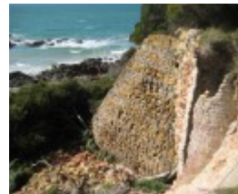
Bell Point Lime Kiln, September 2011
