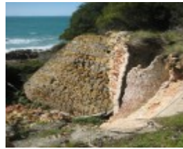
Bell Point Lime Kiln, September 2011
