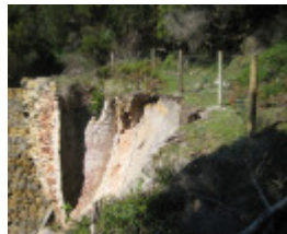
Bell Point Lime Kiln, September 2011
