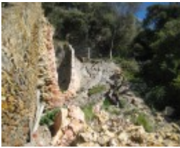
Bell Point Lime Kiln, September 2011
