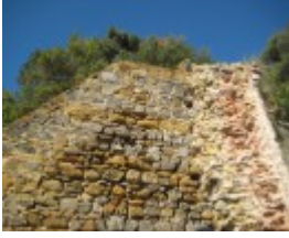
Bell Point Lime Kiln, September 2011
