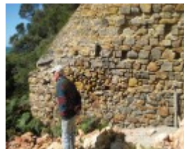
Bell Point Lime Kiln, September 2011
