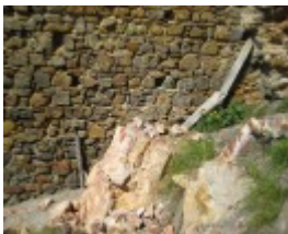
Bell Point Lime Kiln, September 2011
