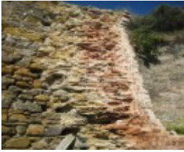
Bell Point Lime Kiln, September 2011
