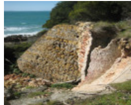
Bell Point Lime Kiln, September 2011
