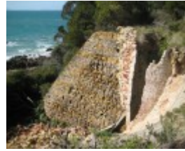
Bell Point Lime Kiln, September 2011
