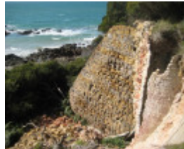
Bell Point Lime Kiln, September 2011
