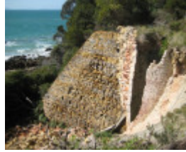
Bell Point Lime Kiln, September 2011
