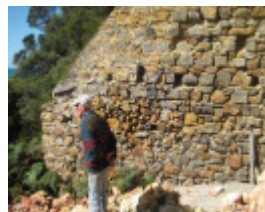
Bell Point Lime Kiln, September 2011
