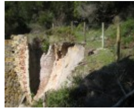
Bell Point Lime Kiln, September 2011
