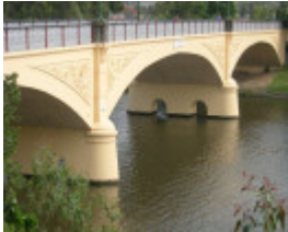
MORELL BRIDGE SOHE 2008
