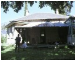
1 residence 64 avoca street south melbourne front view
