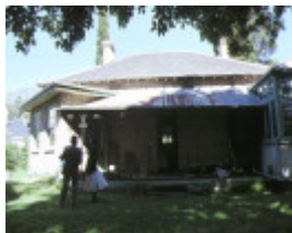
1 residence 64 avoca street south melbourne front view
