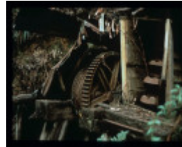
WHITE STAR NO.1 MINE & MACHINERY SITE FEATURE
