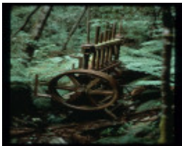
WHITE STAR NO.1 MINE & MACHINERY SITE FEATURE
