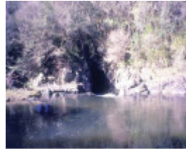
h01990 1 thomson river diversion tunnel entrance
