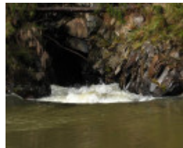
Inlet pool, rock bar and inlet of the diversion tunnel (north end of site)
