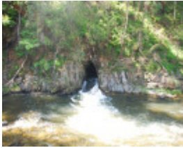
THOMSON RIVER DIVERSION TUNNEL SOHE 2008
