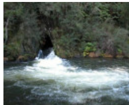
outlet pool at the outlet end of the diversion tunnel (south end of site)
