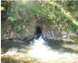
THOMSON RIVER DIVERSION TUNNEL SOHE 2008
