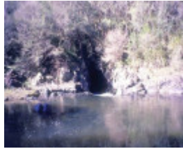
h01990 1 thomson river diversion tunnel entrance
