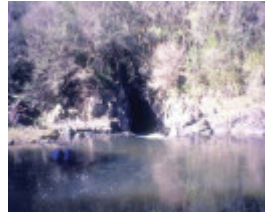
h01990 1 thomson river diversion tunnel entrance
