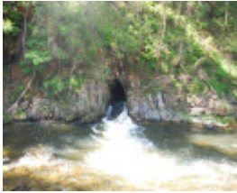
THOMSON RIVER DIVERSION TUNNEL SOHE 2008
