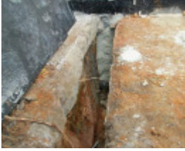
During Photograph - Reference F3856 2015
