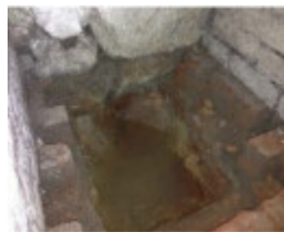
Before Photograph - Reference F3856 2014
