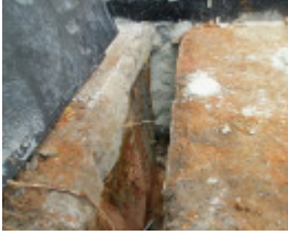
During Photograph - Reference F3856 2015
