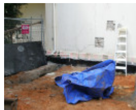
During Photograph - Reference F3856 2015
