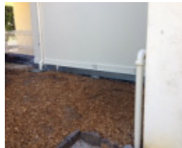
After Photograph - Reference F3856 2016
