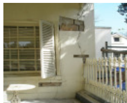
During Photograph - Reference F3856 2015
