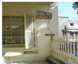
During Photograph - Reference F3856 2015
