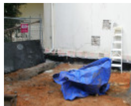
During Photograph - Reference F3856 2015
