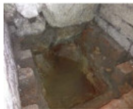
Before Photograph - Reference F3856 2014
