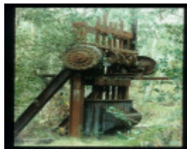
DRY CREEK-HARBINGER BATTERY AND MINE WORKINGS
