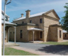
1 beechworth courthouse ford street beechworth front view nov99
