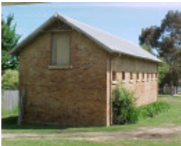
Police Stables Ford Street Beechworth November 99
