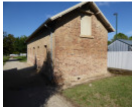
After Photograph - Reference F3879 2016
