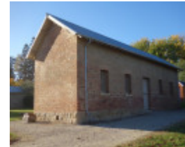
Before Photograph - Reference F3879 2014
