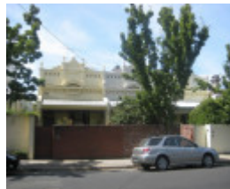
Victorian terrace, Cassell Street
