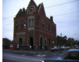
1 former south yarra post office south yarra front view
