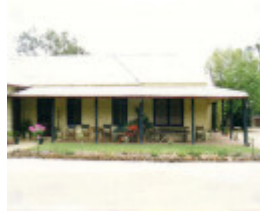
MAW 02 2 - Photograph of renovated early homestead - Shire of Northern Grampians - Stage 2 Heritage Study, 2004
