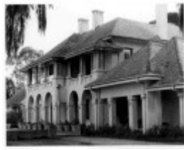
MAW 02 1 - State Library of Victoria, John Collins Collection, Main House before fire - Shire of Northern Grampians - Stage 2 Heritage Study, 2004
