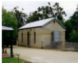
MAW 02 4 - Photograph of rendered brick storehouse - Shire of Northern Grampians - Stage 2 Heritage Study, 2004
