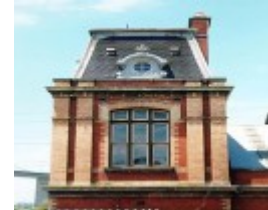
1 former mmbw pumping station douglas parade spotswood tower view aug1987
