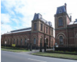
SEWERAGE PUMPING STATION SOHE 2008
