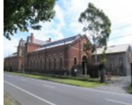
SEWERAGE PUMPING STATION SOHE 2008
