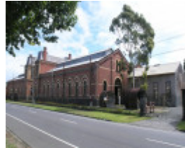
SEWERAGE PUMPING STATION SOHE 2008
