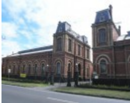
SEWERAGE PUMPING STATION SOHE 2008
