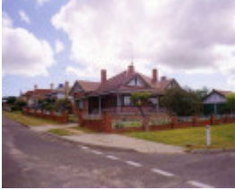
SD 018 - House - 40 Alma Street, ST ARNAUD Shire of Northern Grampians - Stage 2 Heritage Study, 2004
