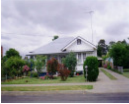
SD 041 - Shire of Northern Grampians - Stage 2 Heritage Study, 2004
