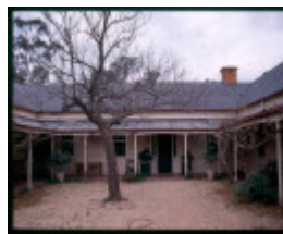
H0305 Tottington Homestead courtyard
