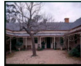
H0305 Tottington Homestead courtyard
