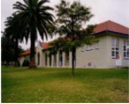
SD 052 - Primary School No. 1646, NORTHERN GRAMPIANS SHIRE
