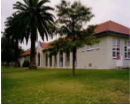
SD 052 - Primary School No. 1646, NORTHERN GRAMPIANS SHIRE
