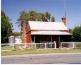
SD 066 - House, 8 Inglewood (Bendigo - St Arnaud) Road, ST ARNAUD
