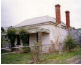
SD 067 - House, 11 Inglewood (Bendigo - St Arnaud) Road, ST ARNAUD
