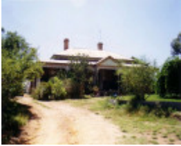
SD 069 - House, Inglewood (Bendigo - St Arnaud) Road, ST ARNAUD
