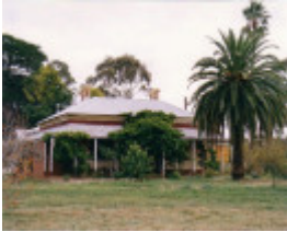
SD 077 - House - 'Burnside', 37-43 Kell Road cnr Reservoir Road, ST ARNAUD
