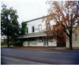
SD 080a - Former Bell and Lorimer General Store, 24 Kings Avenue, ST ARNAUD
