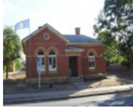
CROWN LAND OFFICE SOHE 2008
