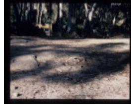
ECHO POINT FOOTINGS
