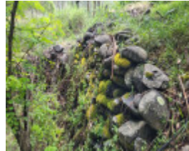
Retaining wall near sluiced ground
