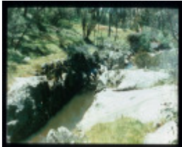
OSBORNE'S FLAT DIVERSION SLUICE
