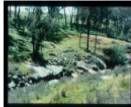
OSBORNE'S FLAT DIVERSION SLUICE
