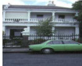
1 residence 8 burnett street st kilda front elevation mar1989
