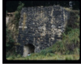
BOGGY CREEK LIME KILNS
