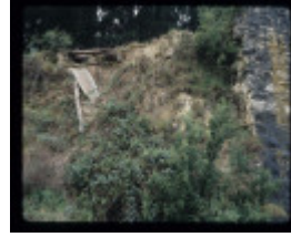
BOGGY CREEK LIME KILNS
