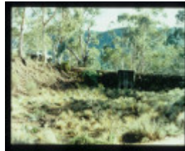
VICTORIA FALLS HYDRO-ELECTRIC POWER STATION
