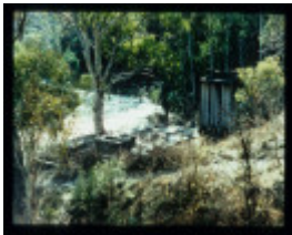
VICTORIA FALLS HYDRO-ELECTRIC POWER STATION
