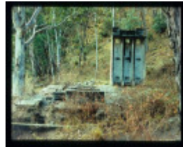
VICTORIA FALLS HYDRO-ELECTRIC POWER STATION
