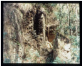
ROSE THISTLE AND SHAMROCK WORKINGS - BOILER SETTING
