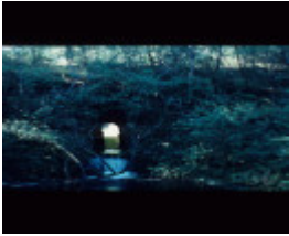
HOUGHTON'S/MCCOY'S FLAT DIVERSION TUNNEL
