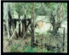
WARDEN BATTERY AND TREATMENT WORKS SITE
