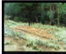
MT HEPBURN COMPANY GOLD TREATMENT WORKS
