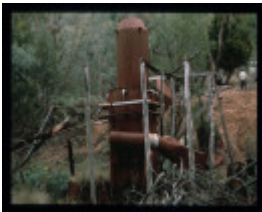
MT HEPBURN COMPANY GOLD TREATMENT WORKS
