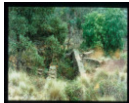
MT HEPBURN COMPANY GOLD TREATMENT WORKS
