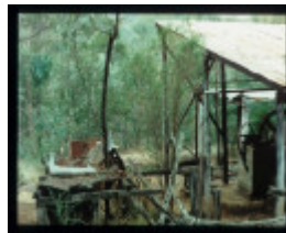
MT HEPBURN COMPANY GOLD TREATMENT WORKS
