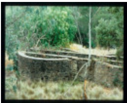
MT HEPBURN COMPANY GOLD TREATMENT WORKS
