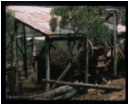
MT HEPBURN COMPANY GOLD TREATMENT WORKS
