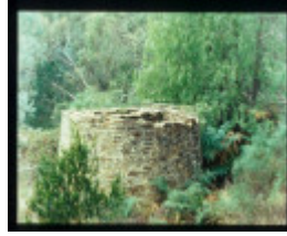
MT HEPBURN COMPANY GOLD TREATMENT WORKS
