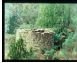
MT HEPBURN COMPANY GOLD TREATMENT WORKS
