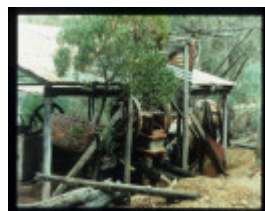
MT HEPBURN COMPANY GOLD TREATMENT WORKS
