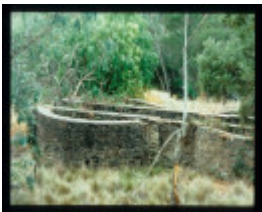
MT HEPBURN COMPANY GOLD TREATMENT WORKS
