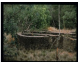
MT HEPBURN COMPANY GOLD TREATMENT WORKS
