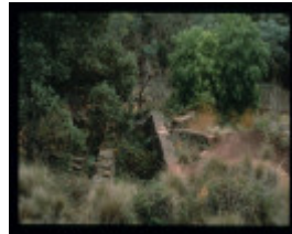
MT HEPBURN COMPANY GOLD TREATMENT WORKS
