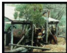
MT HEPBURN COMPANY GOLD TREATMENT WORKS
