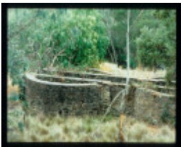
MT HEPBURN COMPANY GOLD TREATMENT WORKS
