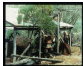
MT HEPBURN COMPANY GOLD TREATMENT WORKS
