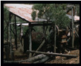
MT HEPBURN COMPANY GOLD TREATMENT WORKS
