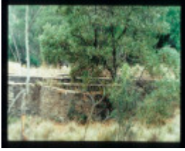
MT HEPBURN COMPANY GOLD TREATMENT WORKS
