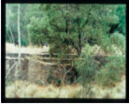
MT HEPBURN COMPANY GOLD TREATMENT WORKS
