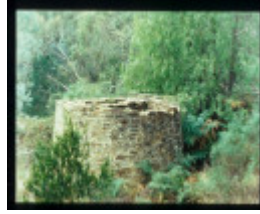
MT HEPBURN COMPANY GOLD TREATMENT WORKS
