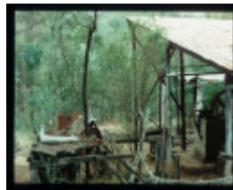
MT HEPBURN COMPANY GOLD TREATMENT WORKS
