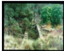
MT HEPBURN COMPANY GOLD TREATMENT WORKS
