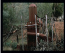
MT HEPBURN COMPANY GOLD TREATMENT WORKS
