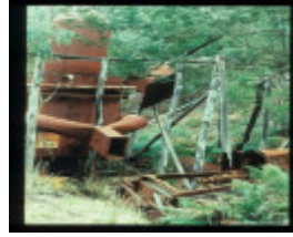
MT HEPBURN COMPANY GOLD TREATMENT WORKS
