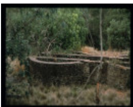
MT HEPBURN COMPANY GOLD TREATMENT WORKS
