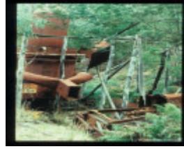
MT HEPBURN COMPANY GOLD TREATMENT WORKS
