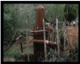
MT HEPBURN COMPANY GOLD TREATMENT WORKS
