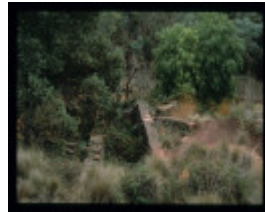
MT HEPBURN COMPANY GOLD TREATMENT WORKS
