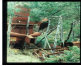
MT HEPBURN COMPANY GOLD TREATMENT WORKS
