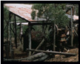
MT HEPBURN COMPANY GOLD TREATMENT WORKS
