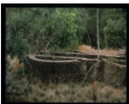
MT HEPBURN COMPANY GOLD TREATMENT WORKS
