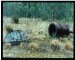
MOUNT MURPHY WOLFRAM TREATMENT WORKS - UPPER WORKS
