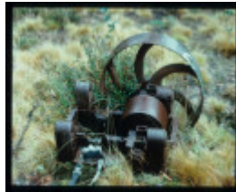
MOUNT MURPHY WOLFRAM TREATMENT WORKS - UPPER WORKS
