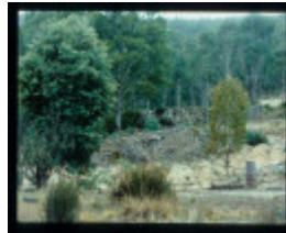
MOUNT MURPHY WOLFRAM TREATMENT WORKS - UPPER WORKS
