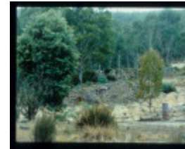
MOUNT MURPHY WOLFRAM TREATMENT WORKS - UPPER WORKS
