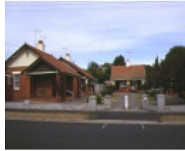
1 alexander miller memorial homes 22 park street geelong complex view apr1997
