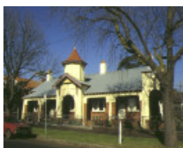
1 alexander miller memorial homes 73 mckillop street geelong front view
