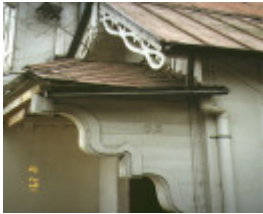
Wattle House Jackson Street St Kilda Entrance Portico Sep 1991
