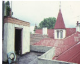
Wattle House Jackson Street St Kilda View of Roof Nov 1985
