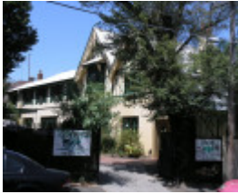
WATTLE HOUSE SOHE 2008
