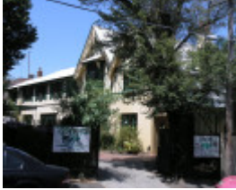
WATTLE HOUSE SOHE 2008
