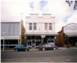
SD 147 - Two-storey building, 31-33 Napier Street, ST ARNAUD
