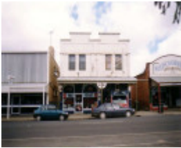
SD 147 - Two-storey building, 31-33 Napier Street, ST ARNAUD
