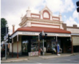
SD/152a - Shop - former 'Victoria Arcade', 53 Napier Street, ST ARNAUD
