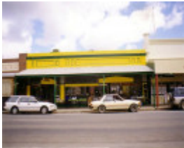
SD 154 - Shop, 'Lyal Eales Store', (former Reeds Store), 59-61 Napier Street, ST ARNAUD
