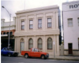
SD 156a - Former Colonial Bank, 62 Napier Street, ST ARNAUD
