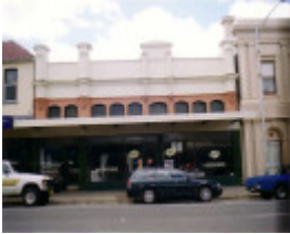
SD 158 - Shops (former Giles Hardware), 64-68 Napier Street, ST ARNAUD
