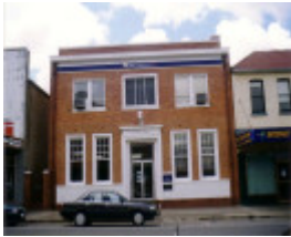
SD 162 - Bank of Melbourne (former Bank of New South Wales), 74 Napier Street, ST ARNAUD
