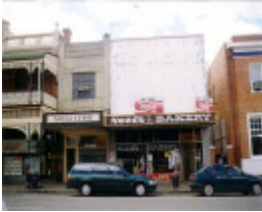
SD 163 - Two-storey building - 'Needs Bakery', 76 Napier Street, ST ARNAUD
