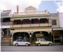
SD 165 - Former Crone's Buildings, 80-84 Napier Street, ST ARNAUD
