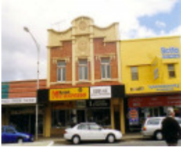
SD 166a - Building - former St. Arnaud Mercury offices, 79-81 Napier Street, ST ARNAUD
