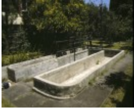
1 sicree family air raid shelter mitford street st kilda elevated view of shelter jan1995
