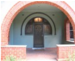
23 Mitford St - entrance porch
