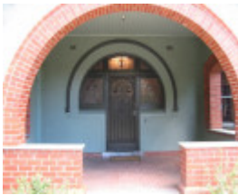
23 Mitford St - entrance porch
