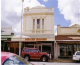
SD 176 - Two-storey building, 106 Napier Street, ST ARNAUD
