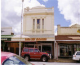
SD 176 - Two-storey building, 106 Napier Street, ST ARNAUD
