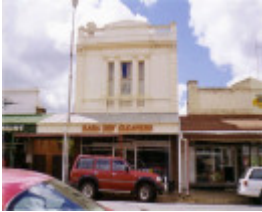
SD 176 - Two-storey building, 106 Napier Street, ST ARNAUD
