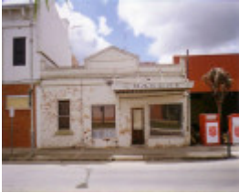
SD 185 - Building - former 'Northend Bakery', 134 Napier Street, ST ARNAUD
